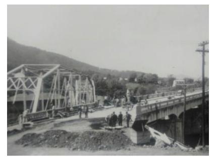
In July of 1937 construction of the current concrete James River Bridge was started with an agreement with the Town under Mayor C. W. Blount to maintain pedestrian access to Pattonsburg via the swinging bridge. In the photo to the left you can see the concrete bridge under construction and the old steel bridge sitting of footers which would be replaced with the new swinging bridge on those same footers. On July 4, 1938, the new bridges were dedicated by former Governor E. Lee Trinkle as speaker.
